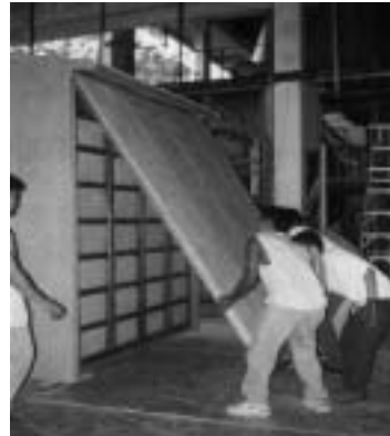
b. Trial run to check roof-to-case connection
