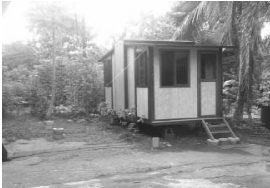
Figure 7. The timber-framed shop-fabricated emergency shelter, complete with false posts, stairs and tie-down straps attached to ground anchorages, currently being service tested at FPRDI
