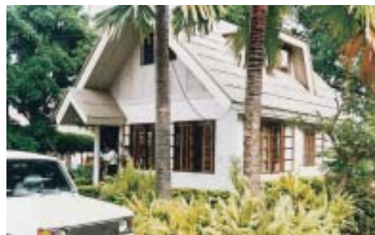
Figure 2. Attractive dwelling in Southern Philippines built using high density wood-wool cement boards
