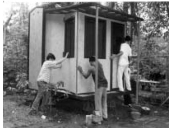
d. The walls are drawn-out from the rigid case, then fixed and locked in place
