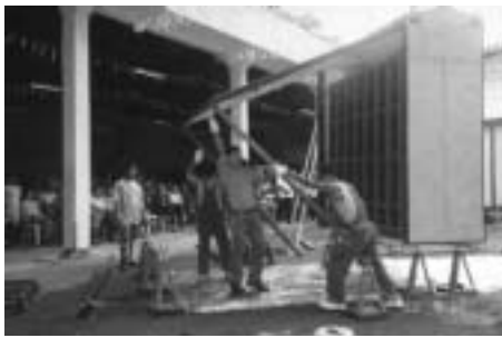
c. Trial run of erecting the second prototype
