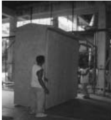
a. Trial fitting of the folded wall, floor and roof components in the case
