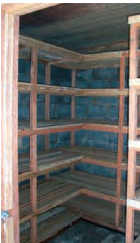
Figure 3.12: Evaporative cooling storage room—a low-cost method of cool storage that doesn't require electricity.
