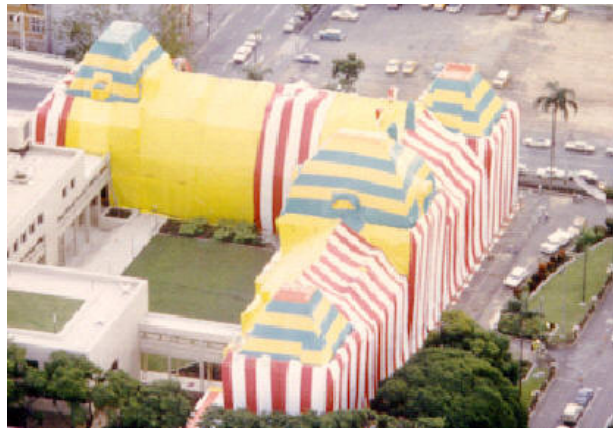
A large building enclosed in gas-proof sheets and fumigated to eradicate an infestation of drywood termites. The enclosure, which took three weeks to build, needed a total of 16 km of 2.5 m wide gas-proof sheeting.
