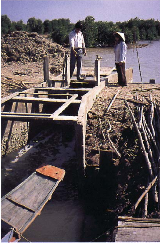
Figure 15. (left) A recently installed, prefabricated, concrete pond gate which are gradually replacing narrow timber gates in the mangrove-shrimp ponds of the Mekong Delta, Vietnam. Photo: Clive Keenan.
