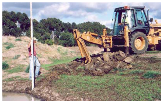
Figure 6. To reduce peak water flow run-off events, off-site buffer dams can be installed. Dam levels are kept low between rainfall events.
