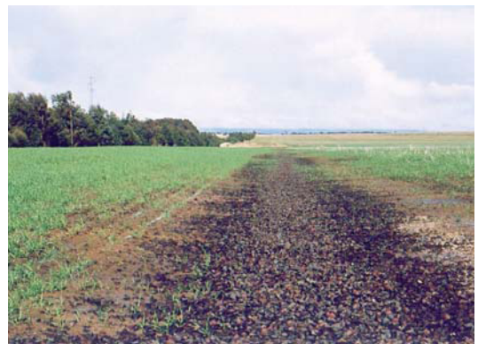
Figure 3. To stop bogging and improve trafficability, collector drains at the ends of the beds can be installed with underground plastic slotted pipes and backfilled with heavy, coarse gravel.
