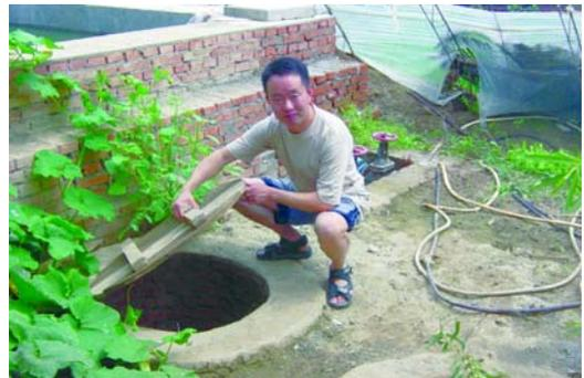
**Figure 7.** (left) Poly-greenhouses with FILTER plots, underlain with a subsurface drainage system; (right) Cheng Xianjun inspecting the drainage sump into which subsurface FILTER drainage water flows. This drainage water (with pollutants reduced below EPA limits) could be reused, or discharged into surface water bodies.
