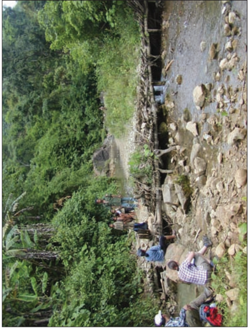
Photo 25.3. A log weir built to divert water to lowland rice fields.
