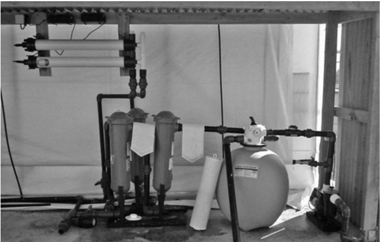
Figure 34. Seawater filtration system.
