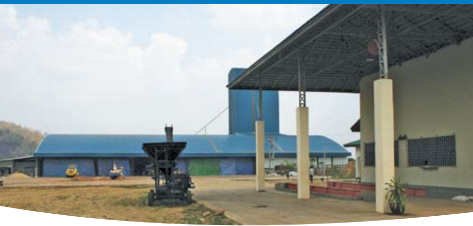
Figure 47. Pailin drying plant, showing weighbridge front right, grain cleaner front left and drying shed in the background
