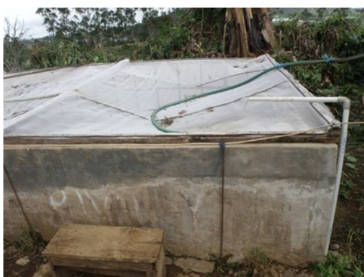
Figure 6.6. Aeroponic water supply holding tank containing unsterilised stream water.
