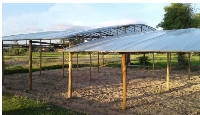
High low plastic roof shelter (timber/bamboo, 2 modules)
