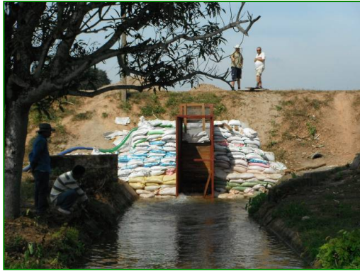
Experimental drop-board weir structure constructed at Nong Teng Fish Hatchery
