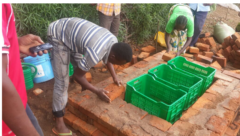
Plate 2: VINESA graduates set up a cooling chamber for prolonging vegetable storage using local available materials (Picture taken by John Macharia).
