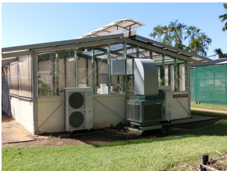
Figure 32: The upgraded glasshouse with two 10 kW air conditioners and a ceiling air vent to keep the day temperatures below 35°C. A similar system is currently being installed at the other end of the building to enable the night temperatures to achieve inductive temperatures (>20°C).
